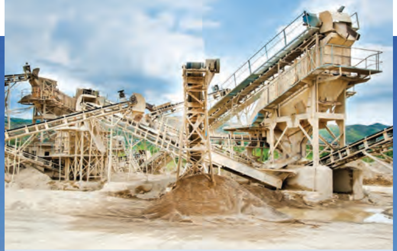
Aggregate, Asphalt and Cement
